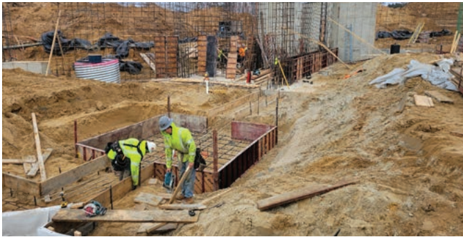
These pictures from March 2022 show crews' work installing footings and foundation walls for the main campus building.
