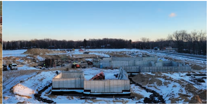
These pictures from March 2022 show crews' work installing footings and foundation walls for the main campus building.
